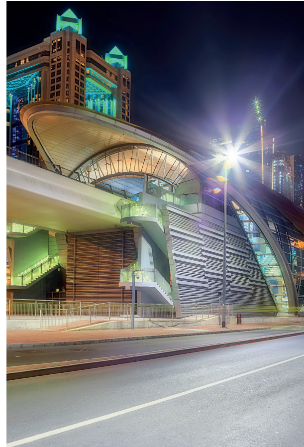
Dubai Burj Khalifa metro station – protected by SteelMaster
